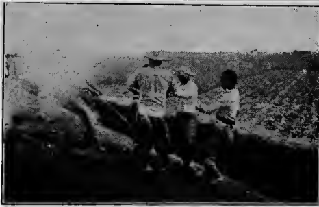
Tamping by use of a "flapper." A "flapper" is a disk of iron or stone weighing about 100 lbs., to which four or more ropes are attached by means of which the workmen swing it up.
