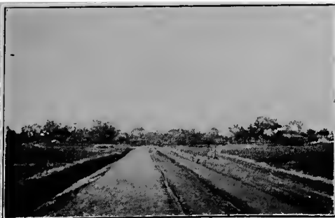
Finished road after some days of illicit narrow-tire cart traffic.
