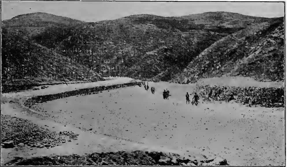
Red Cross road along the river bed. There are miles of retaining walls like this.
