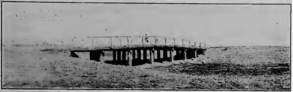
Ancient bridge near Er-Shih-li-pu re-built by the Red Cross. Old railway sleepers were used for the floor and railing.
