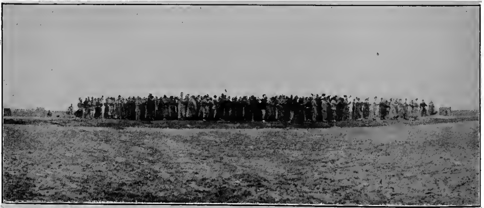
When there was a shortage of tampers, mass treading was found to be fairly efficacious in firming the roadbed.
