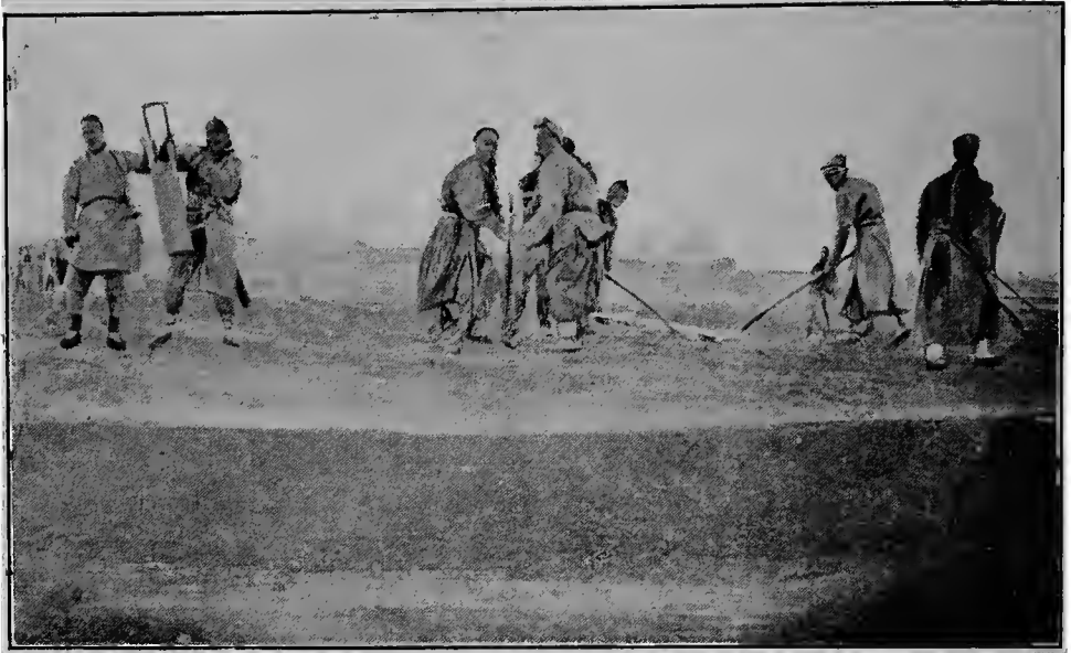
Packing the dirt. Hand tamping was found to be most satisfactory under our conditions.
