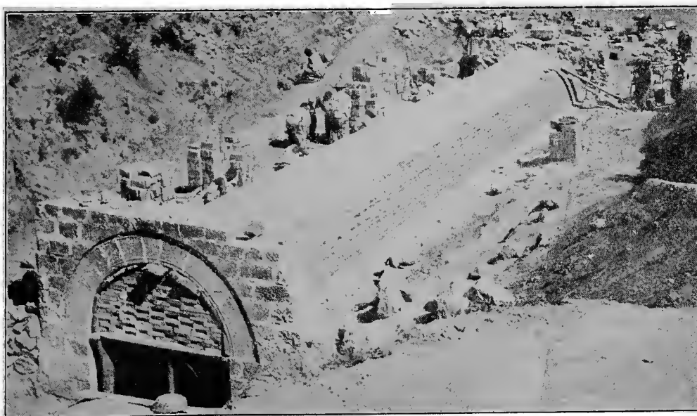
Culvert under construction at Liao Chow.
