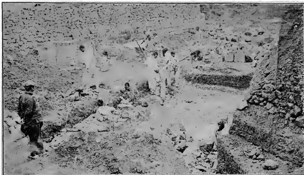
Culvert construction : Preparing foundation.
