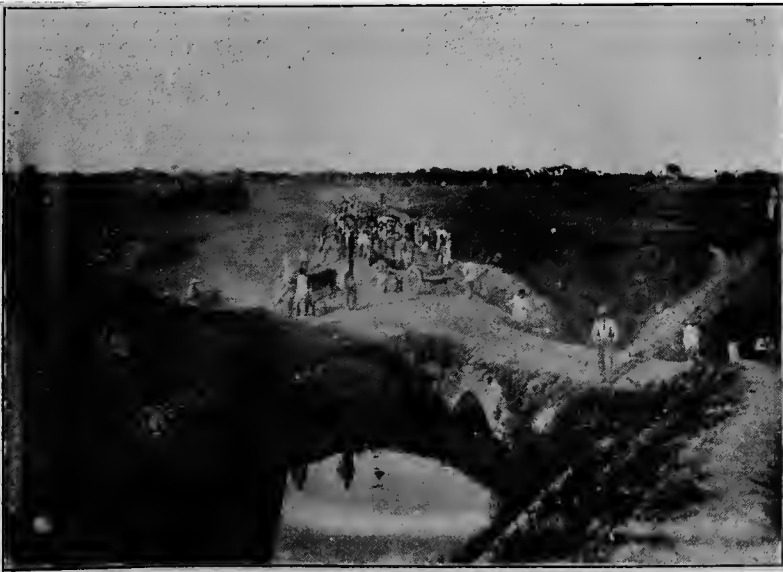
Old Chinese culvert. Later this was extended to full width of the road.
