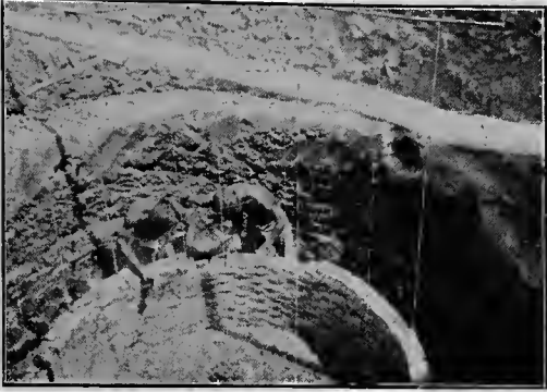
Laying a lining below ground.
