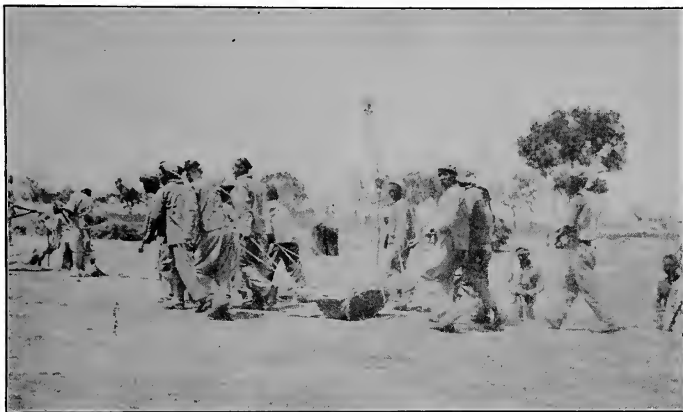
Packing the dirt. This type of roller is too light for satisfactory results.
