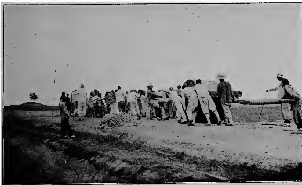
Packing the dirt. This type of roller is too heavy for man power.
