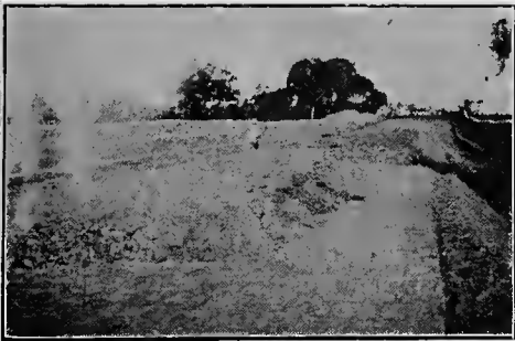
Showing side walls, brick floor laid, and lime-and-clay ready for mixing.
