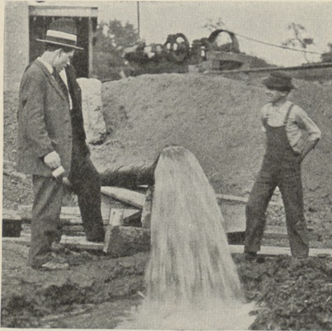
TESTING A DRIVE WELL
