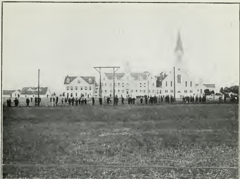
Old Plant—Now Being Replaced
