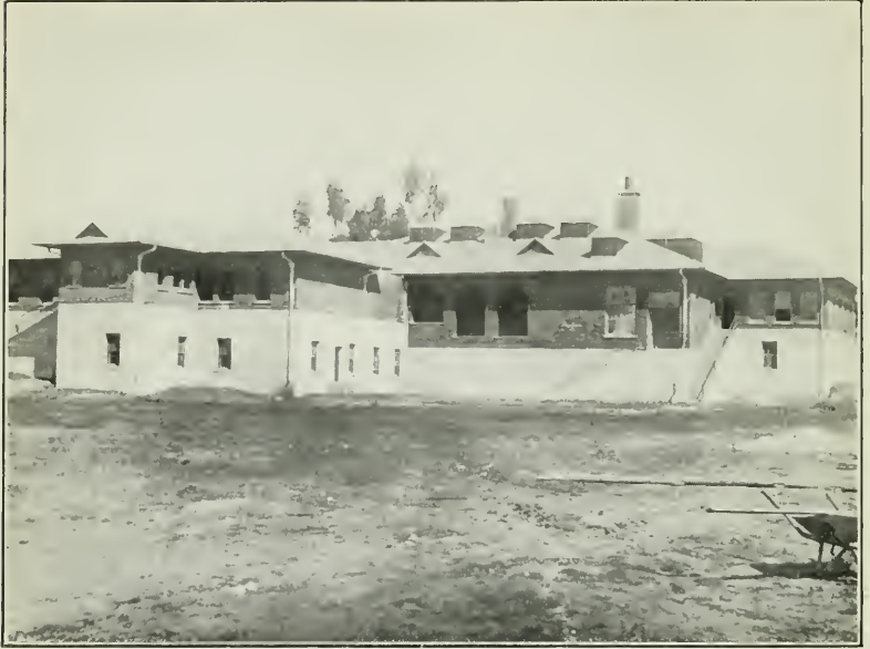
Rear View, Showing Extent of Structure
